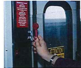
...to break the glass and access the manual door opener.
